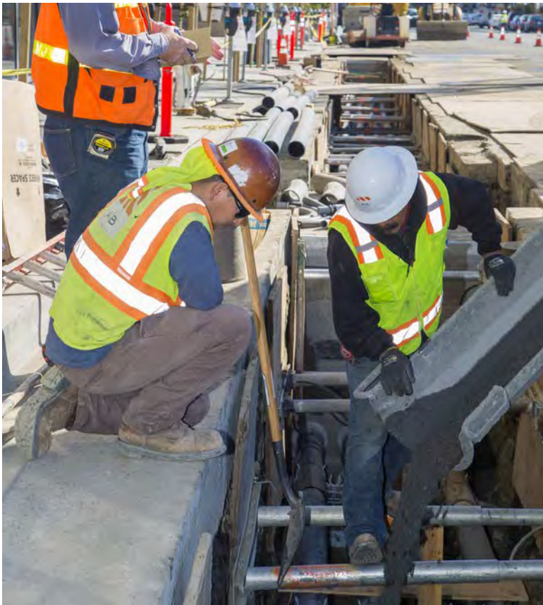
BCTD Project construction in Mission Bay
