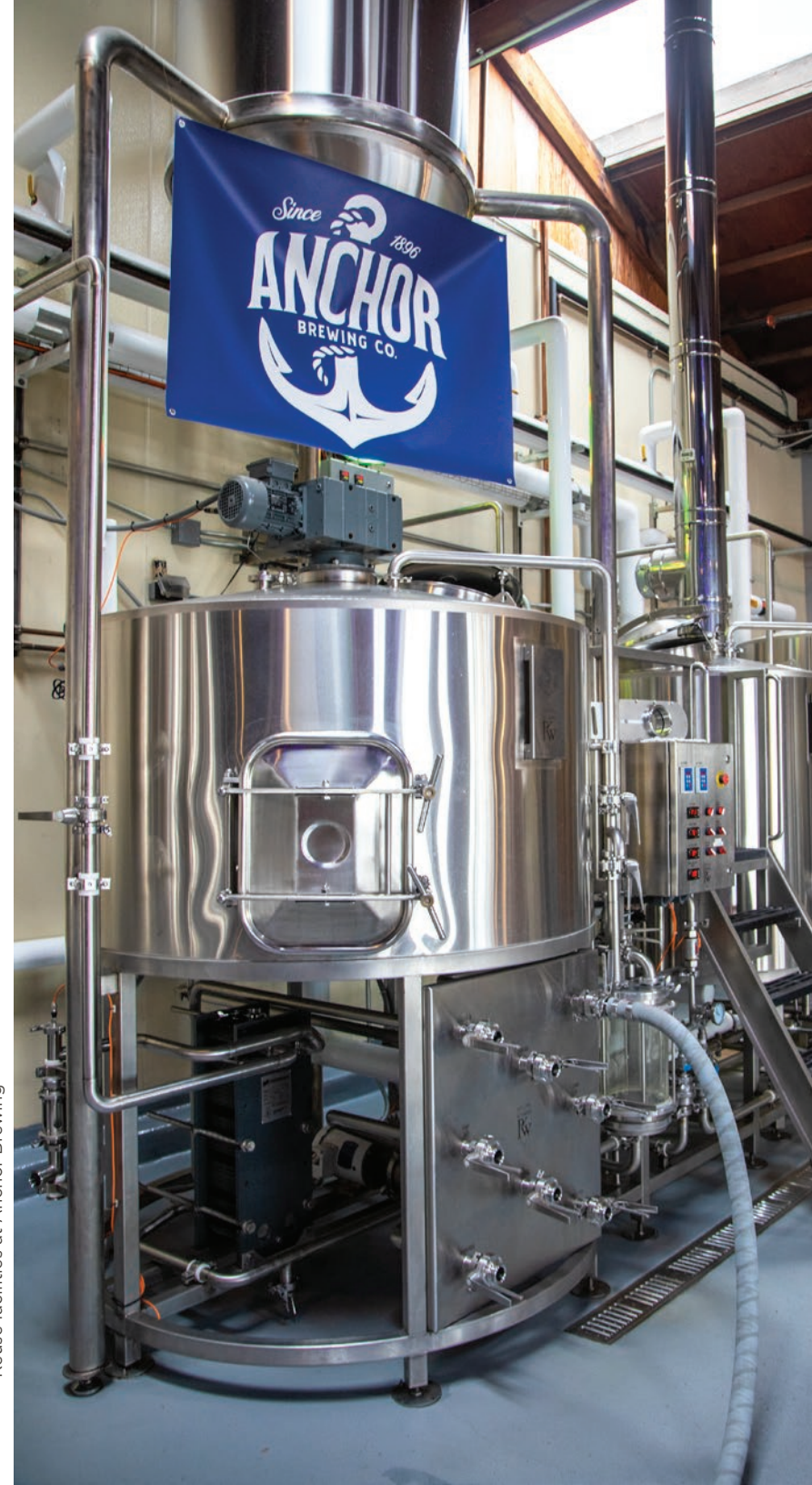
Reuse facilities at Anchor Brewing
