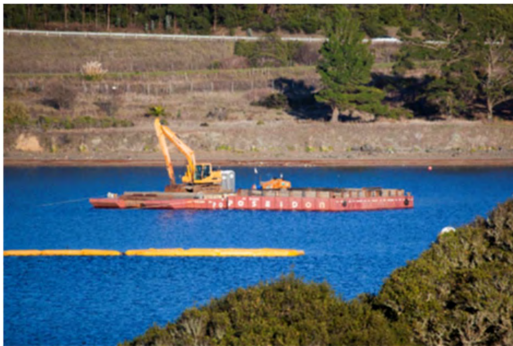
FIGURE 12 - CSSA PROJECT SITE - MARINE CONSTRUCTION
