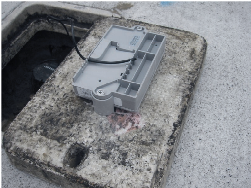
Top: Water meter with transducer. Bottom: Aclara MTU.
