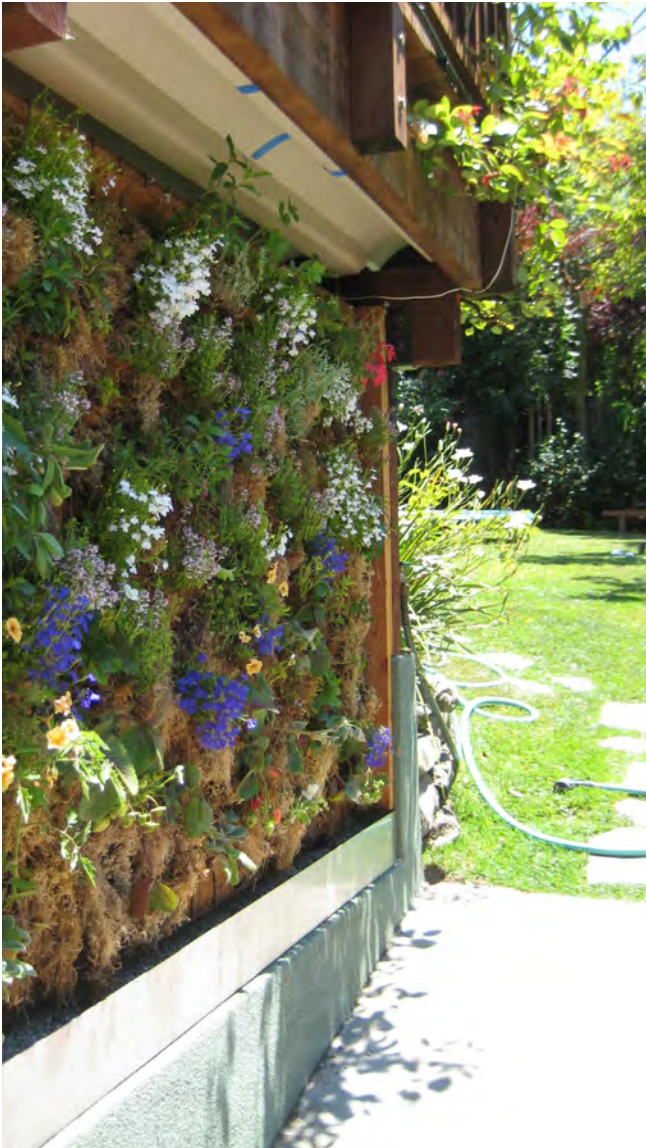
This green wall in San Francisco, CA is irrigated using captured stormwater. Photo: Rachel Kraai
