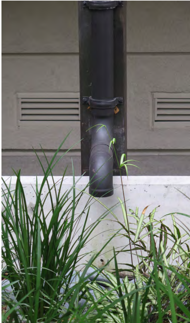
A disconnected roof downspout spills into a bioretention planter. Photo: Krystal Zamora
