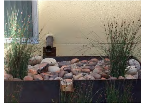
An interior roof drain discharges to a courtyard bioretention planter in San Francisco, CA. This properly designed and permitted stormwater facility is an example of an “approved alternate location” for stormwater discharge. Photo: Polly Perkins
