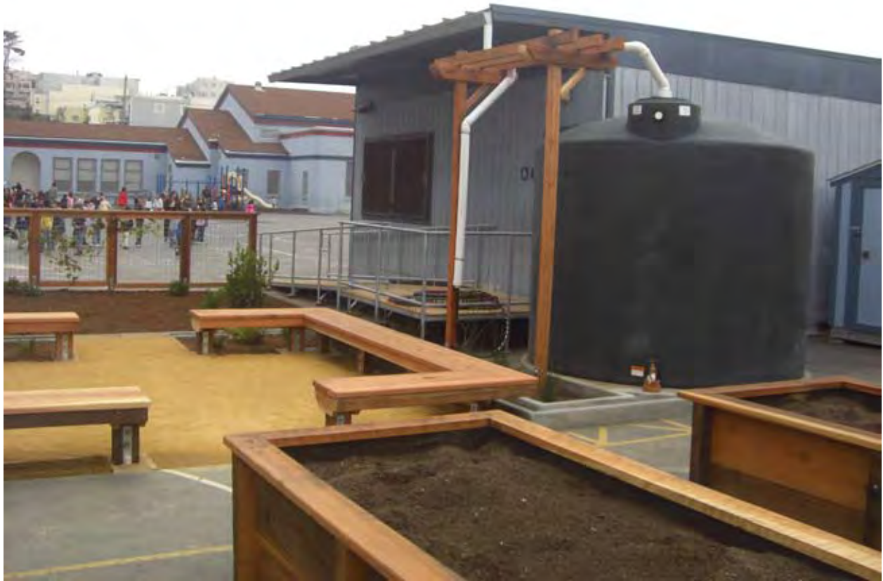
Lafayette Elementary School Rainwater Garden and Cistern, SFUSD
